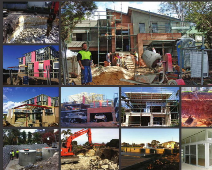
These images Tullipan Homes under construction
